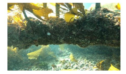
Cables are laid across the top of rock outcrops in the water, or cut into rock channels on the shore, this cable has marine growth on the PE sheath
